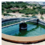
Sewage Treatment Plant (STP)
